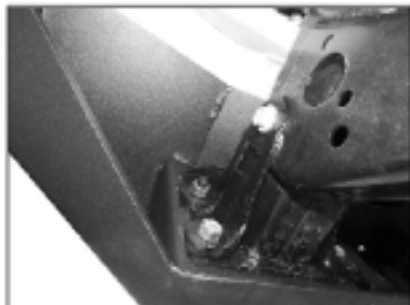
[ Fig 12] Driver/left side of Bumper installed on JL model
